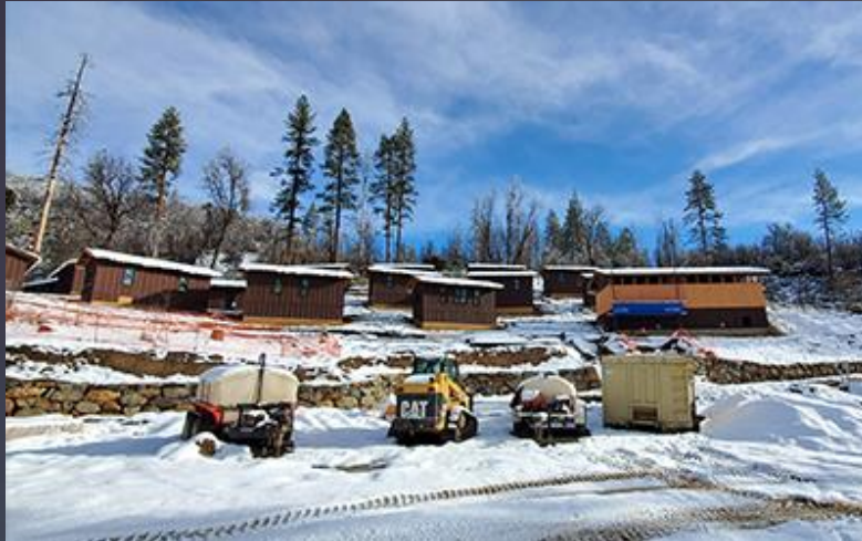
BTC Staff Cabins
